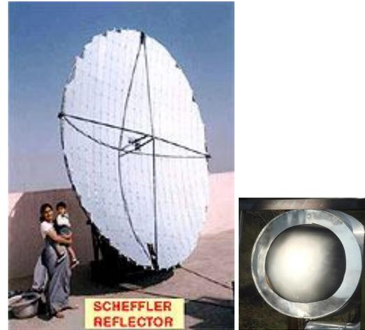
**Figure 8.** Standing Scheffler solar primary and secondary reflector
